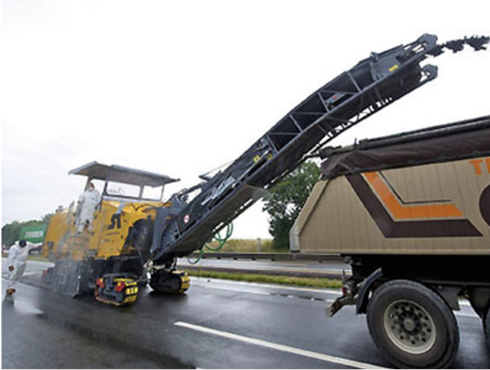
Fig. 5.7 Rehabilitation of the pavement of road under contract [8]
