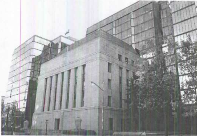
Photograph 1: Bank of Canada building, Ottawa (Photo: William P. McElligott / Bank of Canada)
