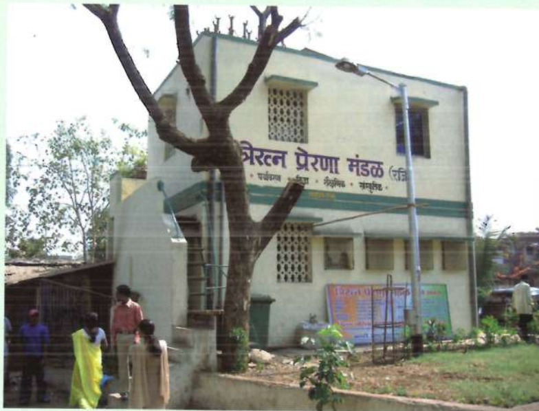
Plate 11.5 An Alliance-built toilet block, Khotiwadi, Mumbai, India. Credit: Colin McFarlane.
