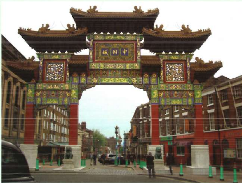
Plate 5.5 The Chinese Arch in Liverpool, UK.
