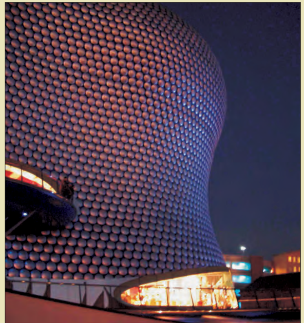
Selfridges Store, Birmingham's Bullring, designed by Future Systems
