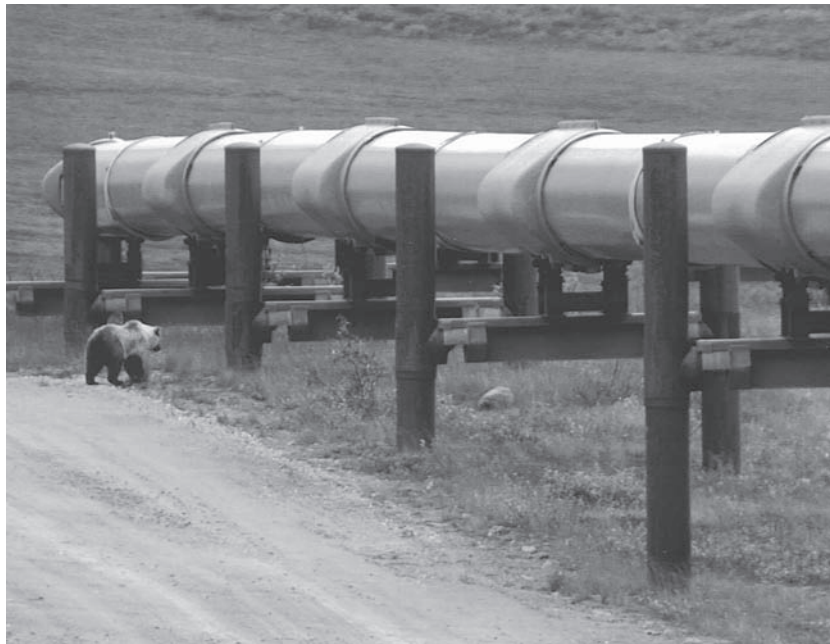
Young grizzly bear at construction site—Atigun section of TransAlaska Pipeline.
