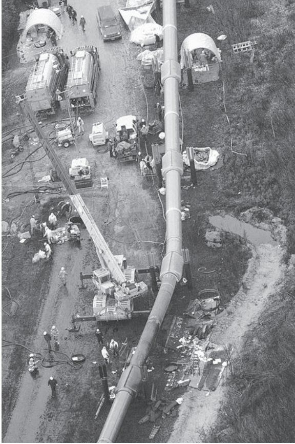
Repairing and maintaining the Pipeline requires constant vigilance.
