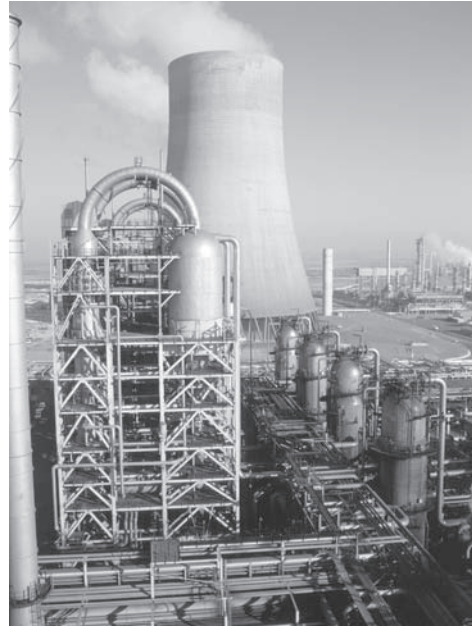
Benfield facility, with columns at the left and right.
