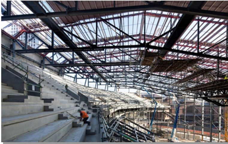
Figure 52.15 Arena during construction
