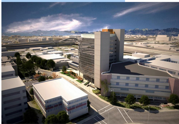
Figure 52.5 PCP tower adjacent to the existing hospital
